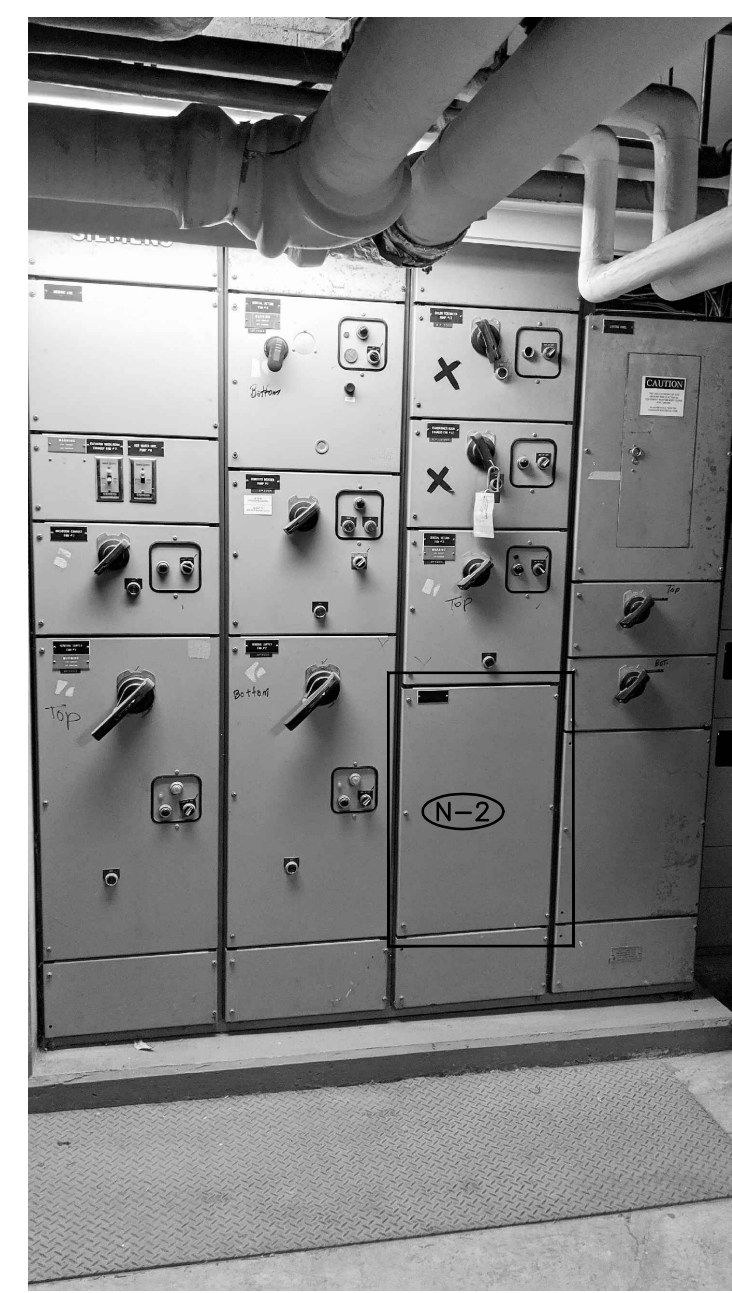
1 EXISTING MOTOR CONTROL CENTER 'MCC AA' INSTLLATION PHOTO E-7.1 SCALE: NTS
